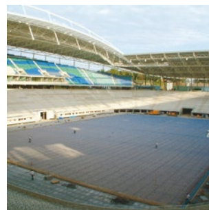
Undersoil pitch heating
